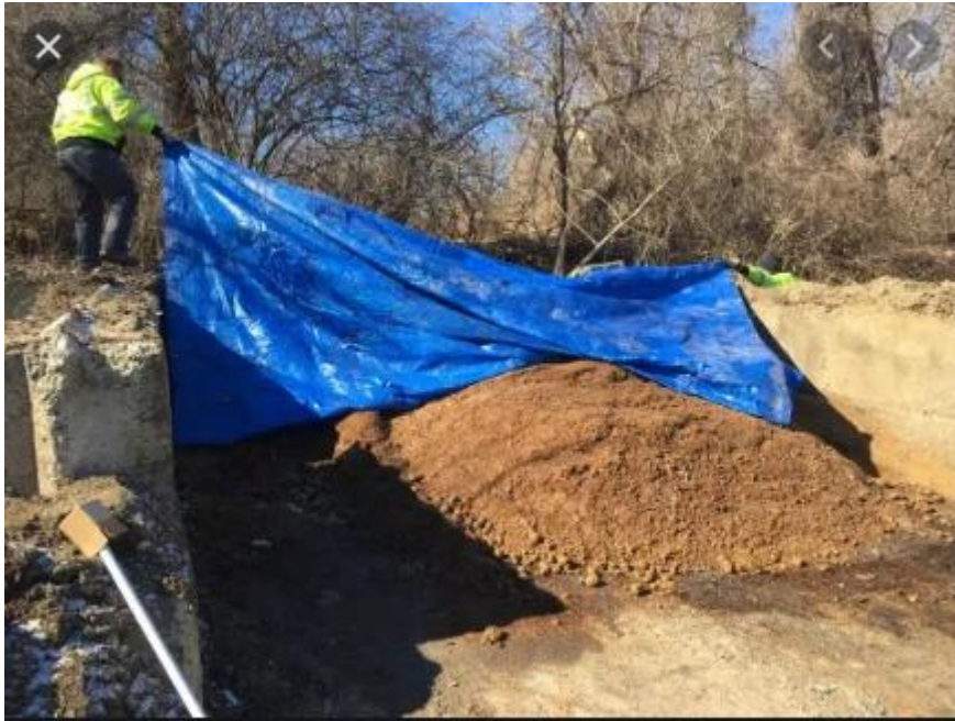
Figure 3.3.1.2.3: Typical impermeable membrane used to dry store topsoil on site.
