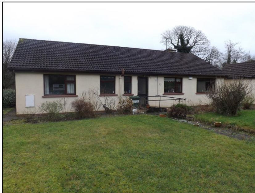
Photo of Rear Elevation
